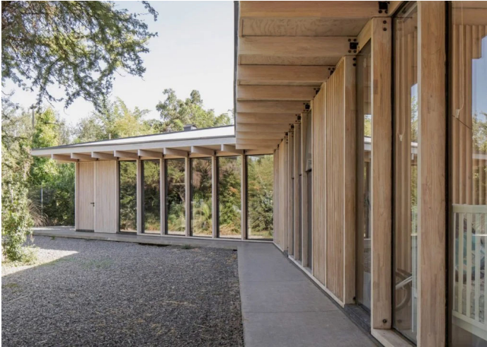
MasFernandez Arquitectura tops Chilean home with triangular skylight
