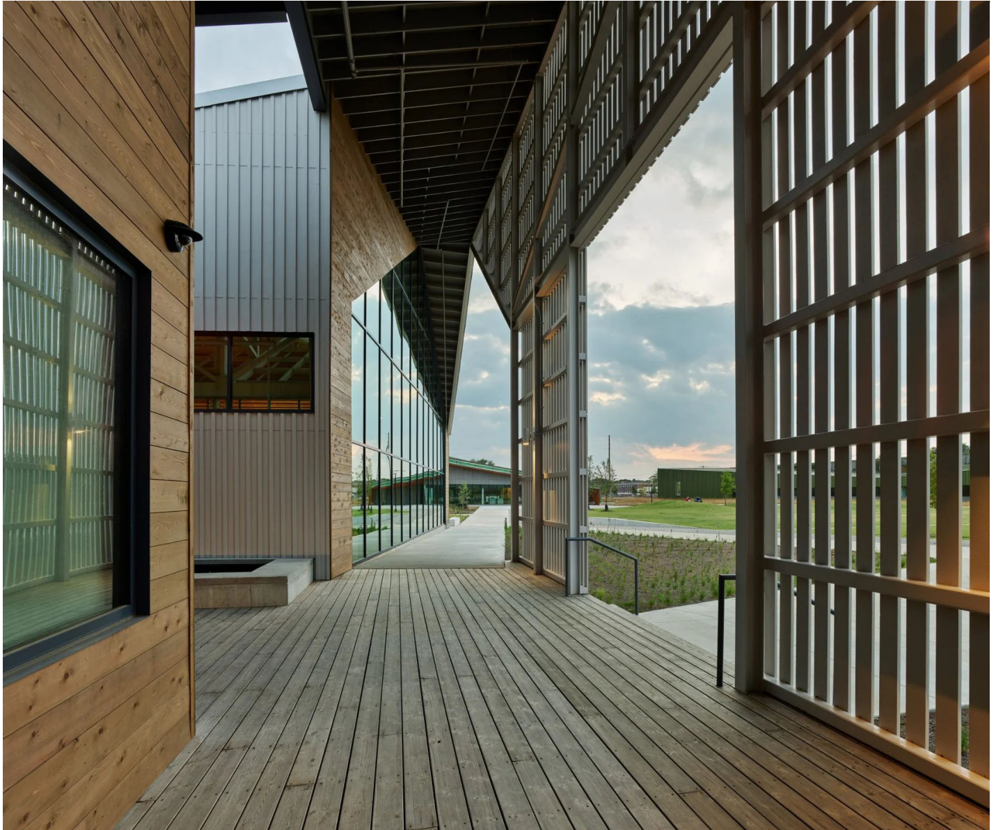
Facades are clad in shiplap cedar siding. Photo is by Tim Hursley
